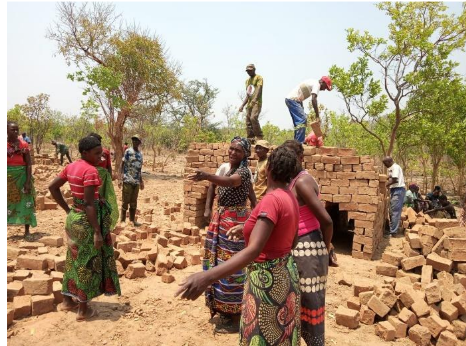
Community members curing bricks at Chaola CS for construction of a classroom block
